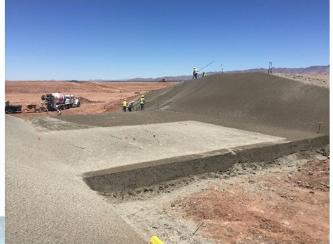
The partially completed spillways. Photo by Granite Construction
