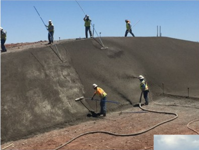
Construction crew working on the spillways. Photo by Granite Construction
