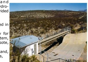
Flow in the main channels on the Walnut Gulch Watershed is measured at 11 gaging stations. Eight of the main tributaries are gaged, and three flumes such as the one in the photo on the left measure flow in the main Walnut Gulch channel.
